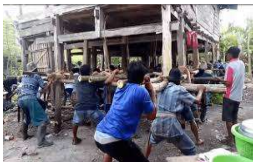
Figure 3: Technical preparation using bamboo and hardwood supports
